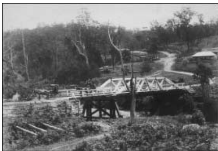
• Dignam's Creek truss bridge, finished in 1893, superseded earlier bridges in the Cobargo county.
