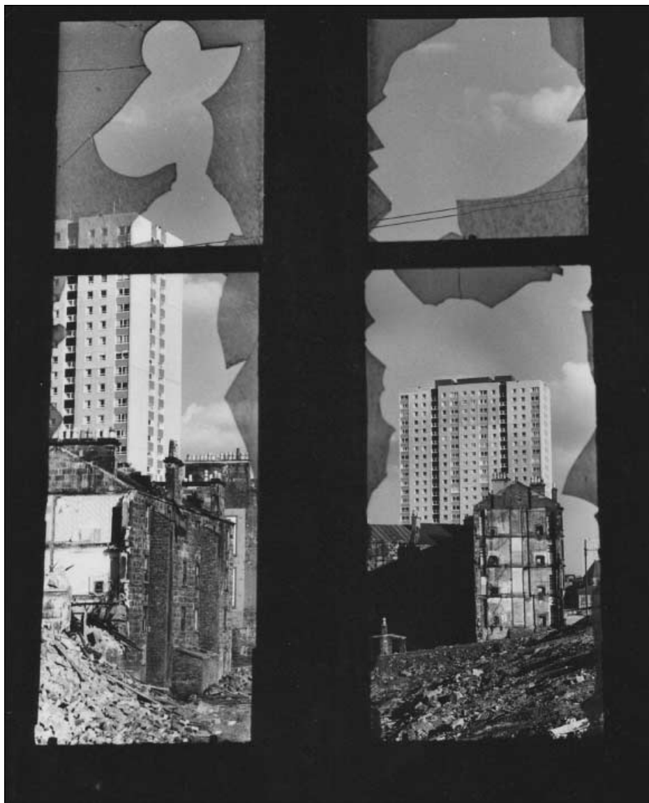
• Stark view in Glasgow 1980 (1970).
