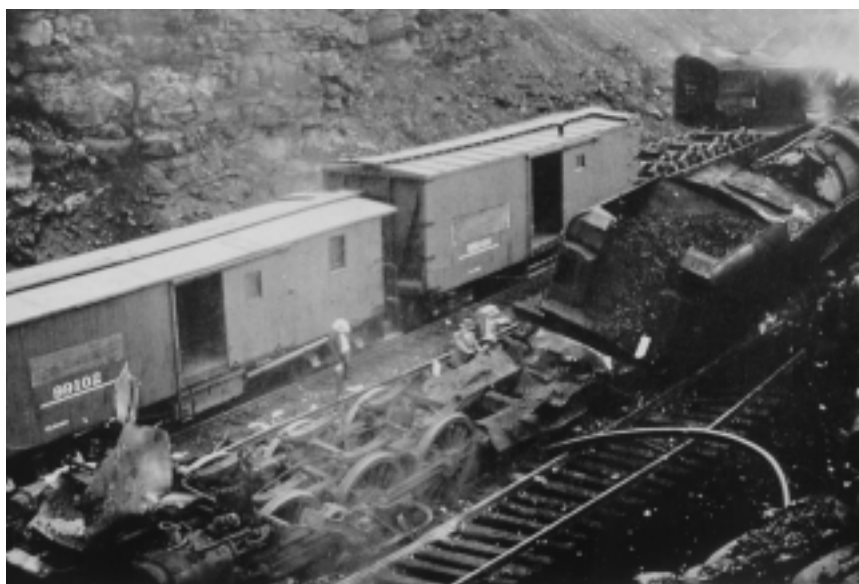
Figure 8 Boiler explosions, although fewer in number, continued to plague steam locomotives . . .
