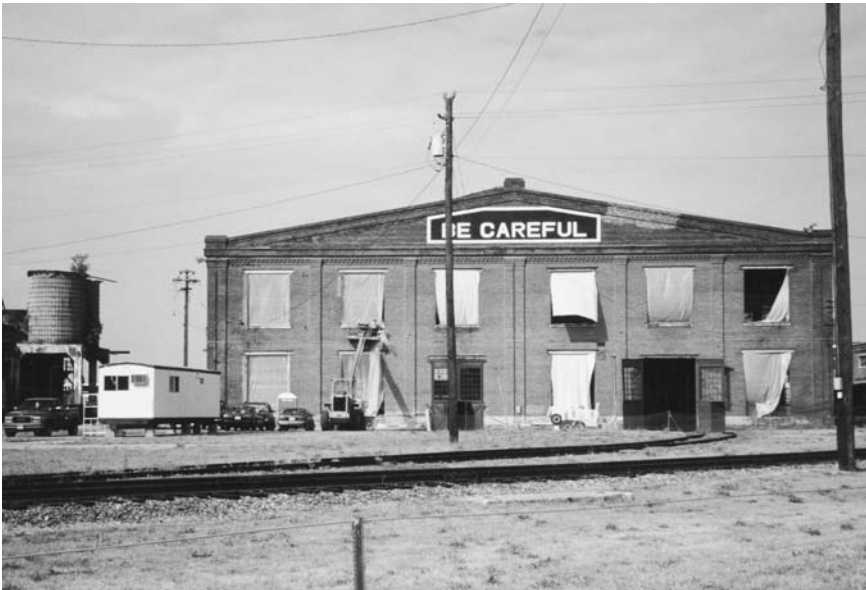
Plate 2 The Back Shop in the process of restoration
